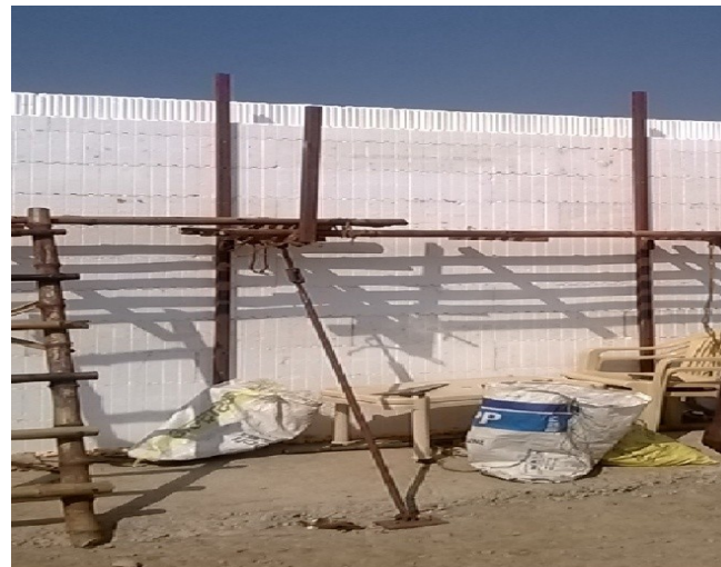
4. ICF wall showing wooden plank walkway on Trestles
