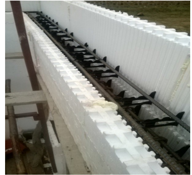
5. ICF wall final layer - with steel ring beam
