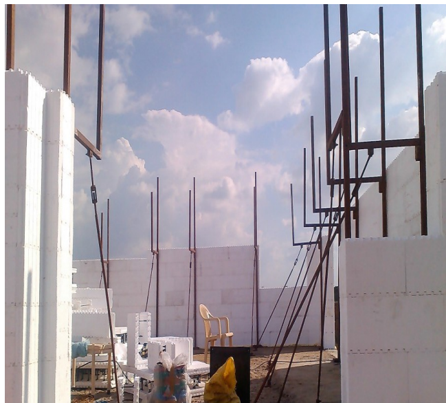
3. ICF wall showing fixing of steel trestles
