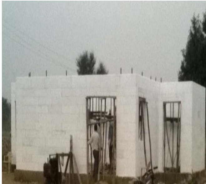
1. The ICF wall with openings for doors & windows
