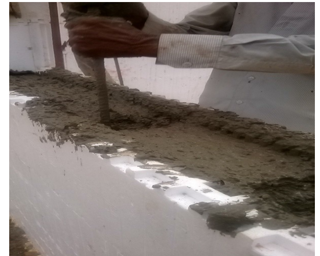
6. Concrete poured in the formwork
